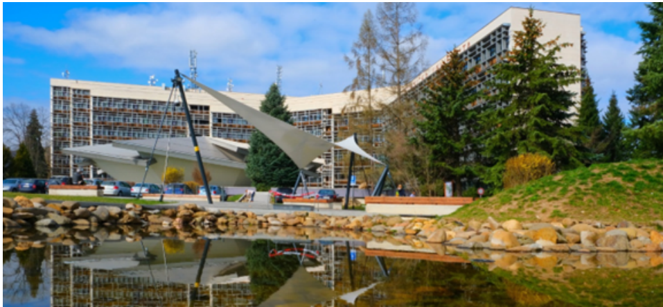
Figure 52 TUZVO main building
