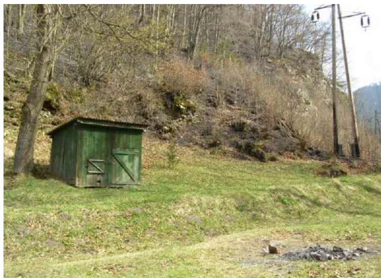
Figure 84 View of the location of the fire in the locality of Staré Hory in 2011 (Source: District Directorate of FRS in Banská Bystrica)
